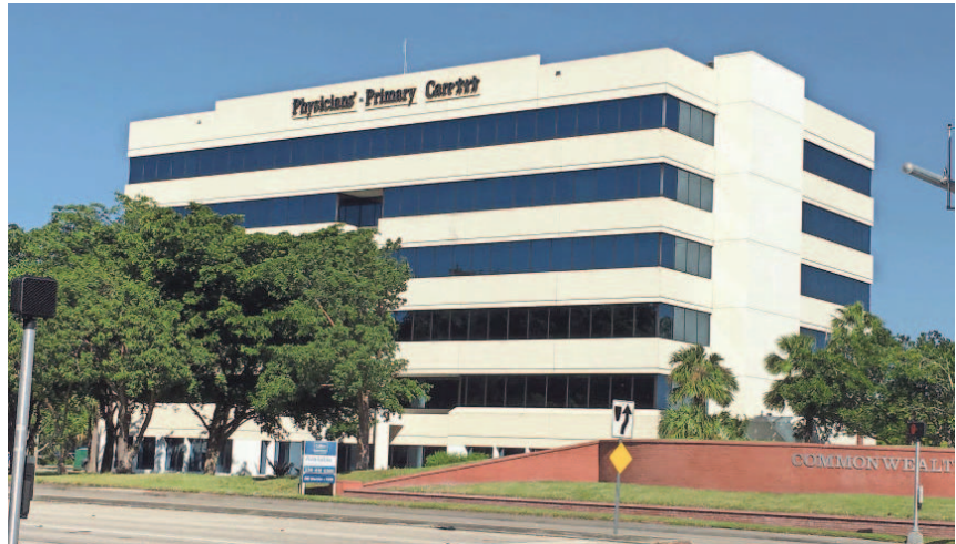
The new administrative offices of Physicians' Primary Care of Southwest Florida in Fort Myers. SPECIAL TO THE NEWS STAR
